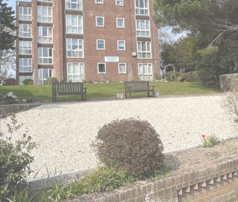
NEW BENCH AND LANDSCAPING AT LANSDELL COURT
